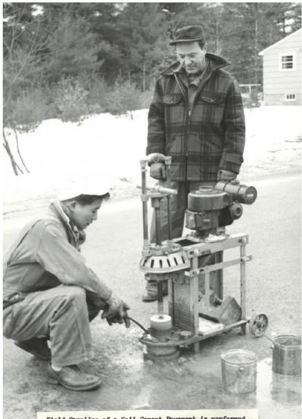
Field Sampling of a Soil-Cement Pavement is performed by laboratory personnel as part of a research project.
