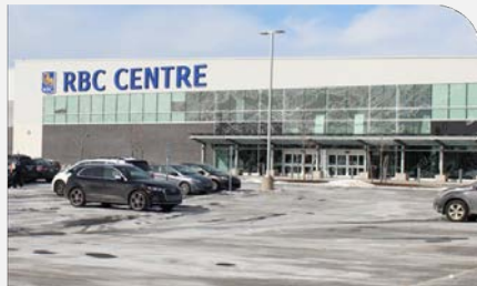
Halifax, NS – RBC Centre Concrete Producer: Quality Concrete CO 2 Saved: 90.7 tonnes
