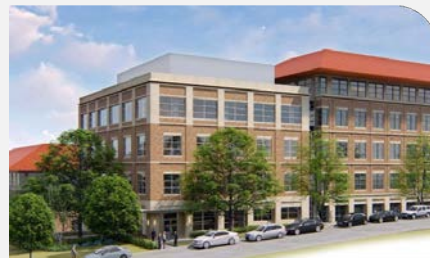
Austin, TX – UT Seay Expansion Concrete Producer: Lauren Concrete CO 2 Saved: 21.5 tonnes
