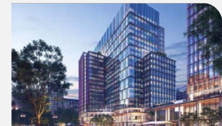
Arlington, VA – Amazon HQ2 Concrete Producers: Miller & Long, Vulcan Materials CO 2 Savings Estimate: 1,043 tonnes
